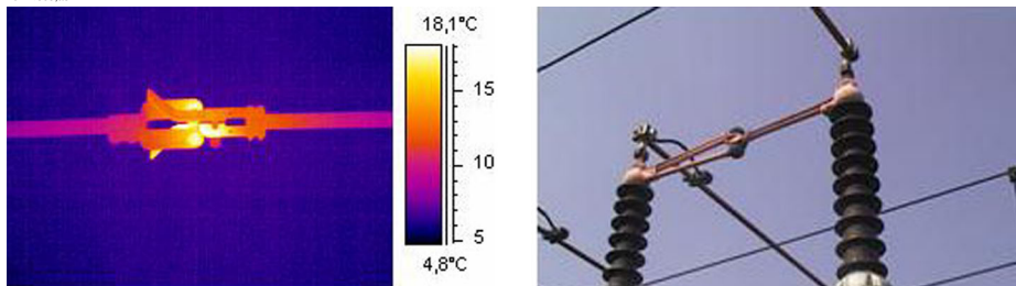
Figure 7.17 Overheating in a circuit breaker
