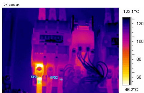
Figure 7.9 An infrared image of indoor electrical equipment (2)
